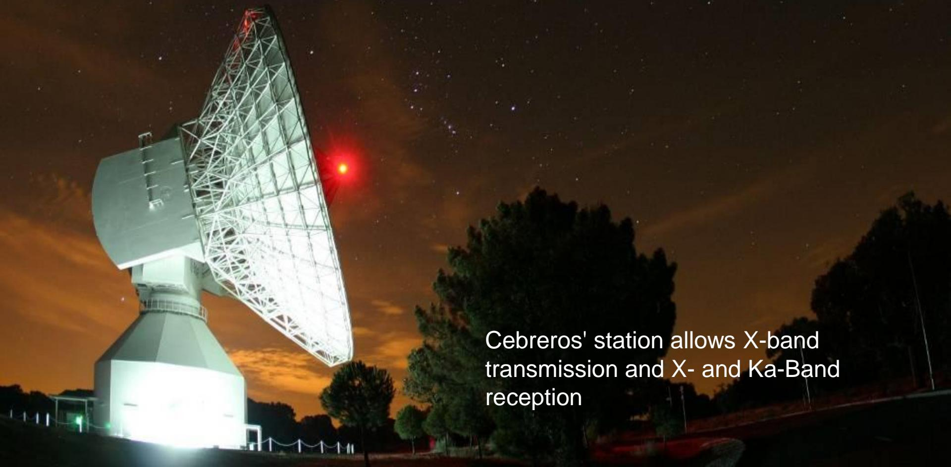
Cebreros' station allows X-band transmission and X- and Ka-Band reception
